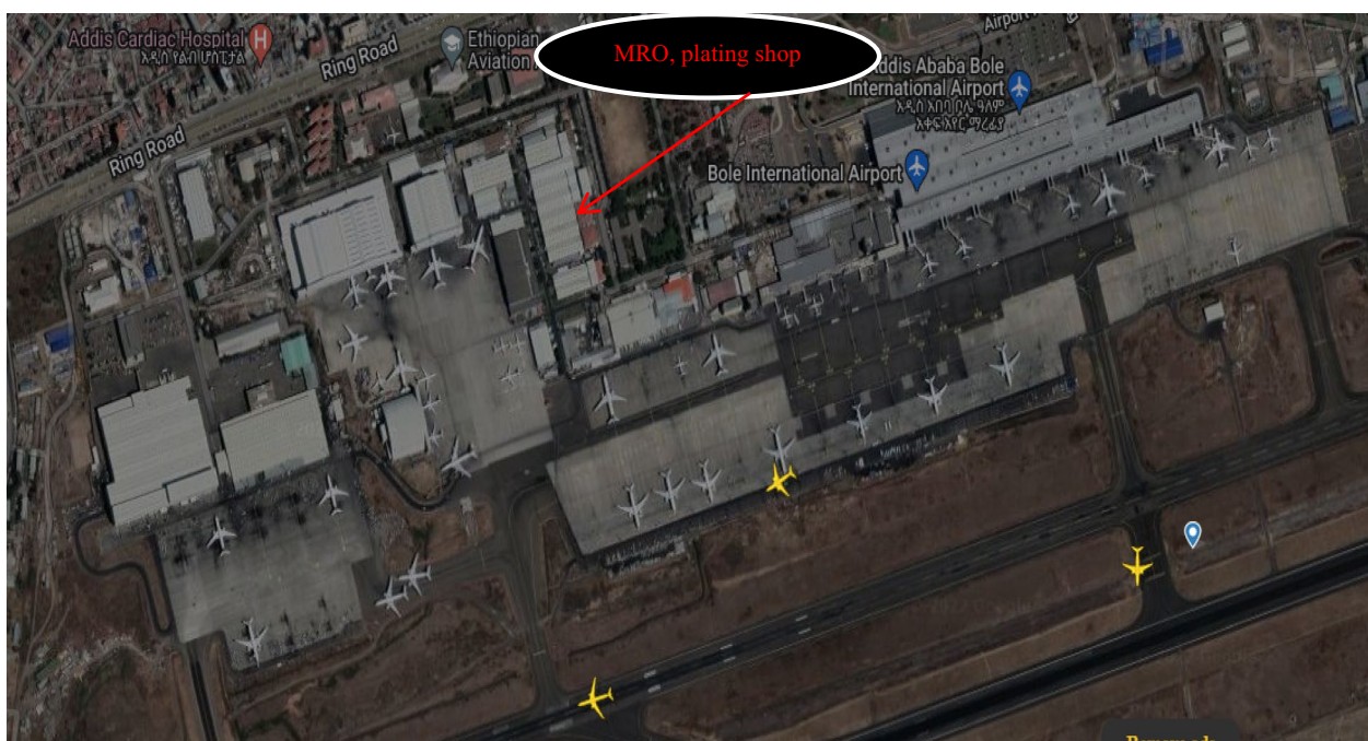
Fig. 1 Ethiopian airlines MRO, Plating Shop location at the Bole international airport
